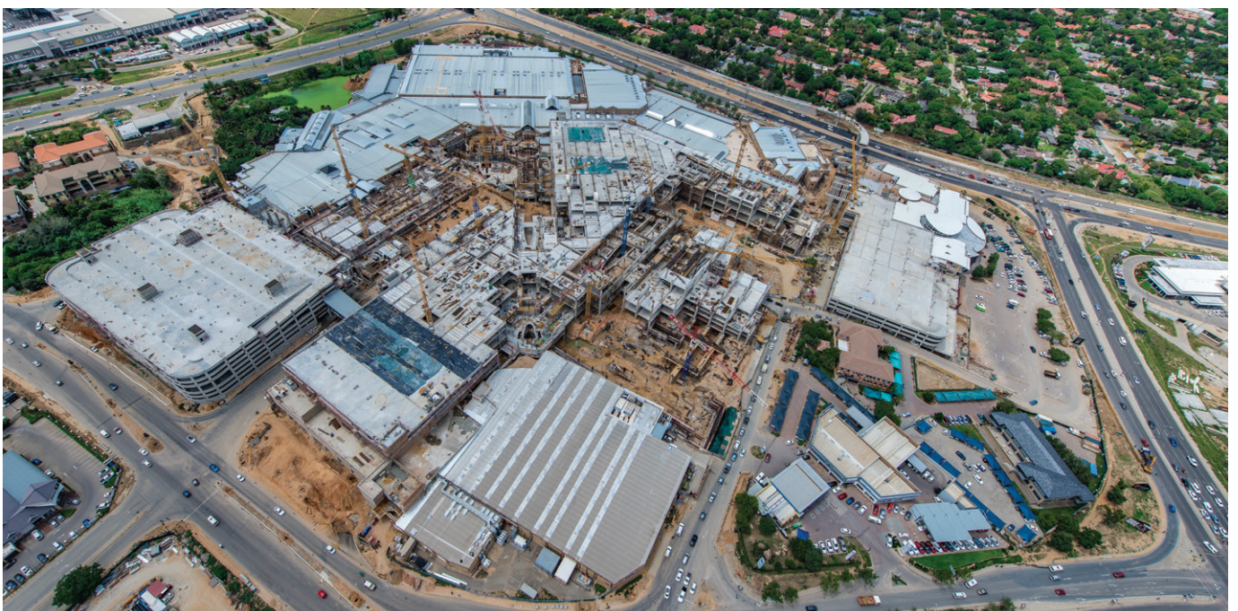
Figure 1: Aerial photo of Fourways Mall Redevelopment.
